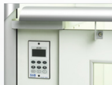
Control and alarm panel for fan fail and sash high warning
